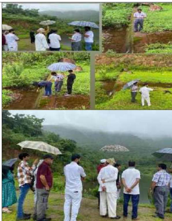
On field measurement and seeing the condition of dam.
