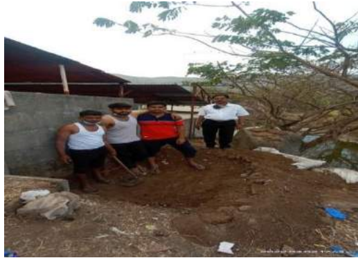
CONSTRUCTION OF COMPOST PIT
